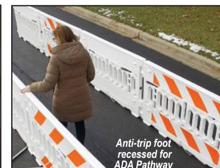
Create ADA Compliant Pedestrian Pathway
