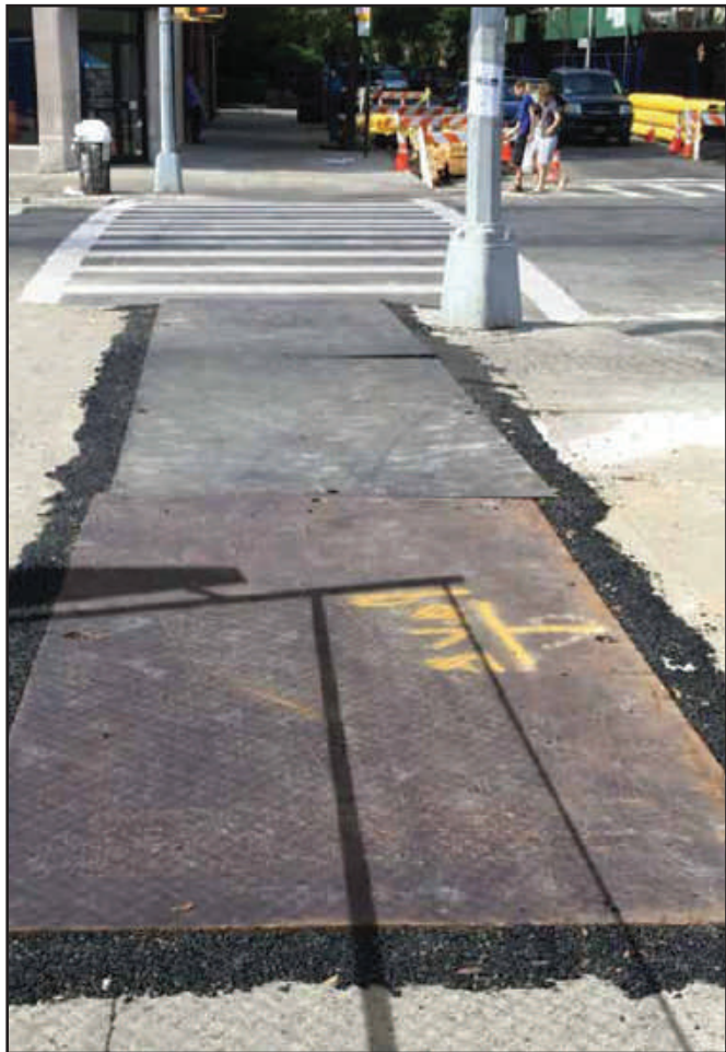
Steel Plates with Cold Patch
