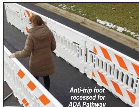
Create ADA Compliant Pedestrian Pathway
