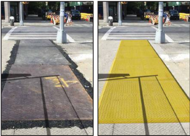
Steel Plates with Cold Patch Plasticade Trench Covers
