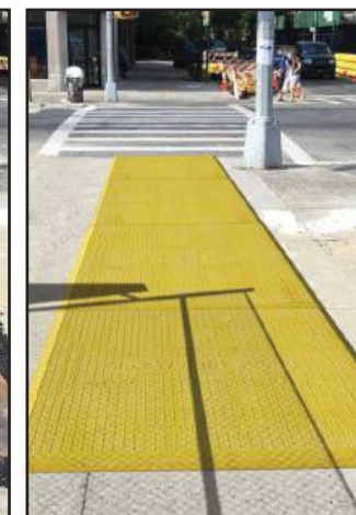
Plasticade Trench Covers
