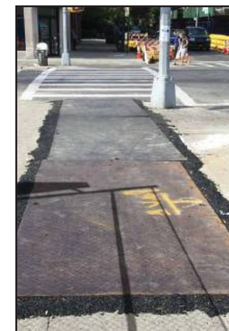
Steel Plates with Cold Patch
